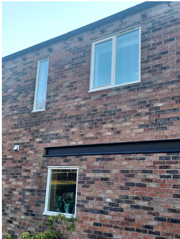
Figure 1 - Typical existing windows and single door
